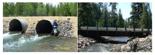
Undersized, paired culverts on Arrastra Creek near stream-mile 3.3 replaced with a free-span bridge in 2005.
