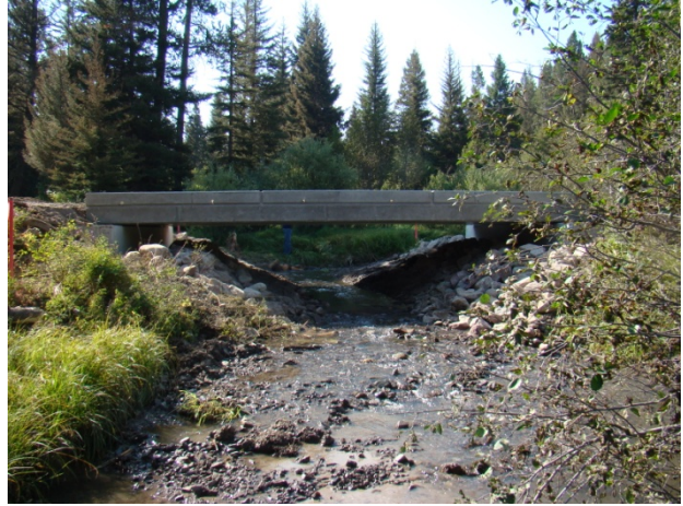
Historic undersized culverts in the Sauerkraut drainage upgraded with free-span bridges to accomodate fish passage.
