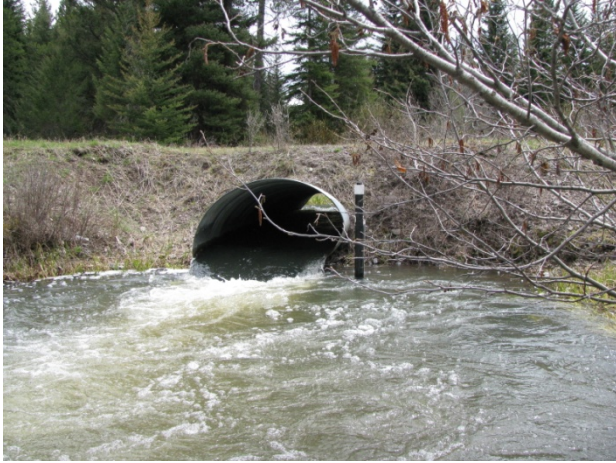
Historic undersized culverts in the Sauerkraut drainage upgraded with free-span bridges to accomodate fish passage.
