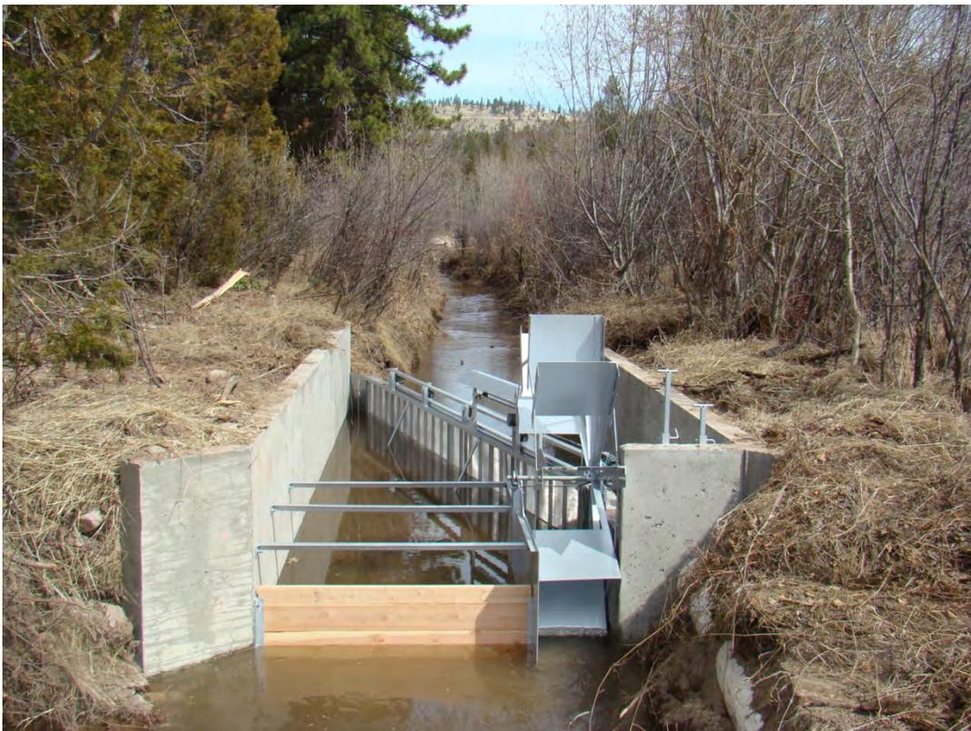
Photos 3-4: Newly installed log vane and self-cleaning paddlewheel fish screen.
