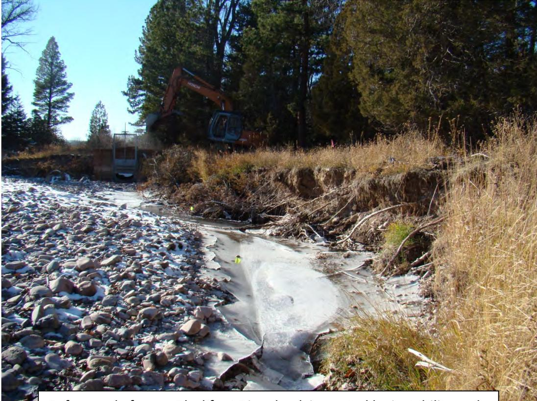
Before and after on Blackfoot River bank impacted by instability and erosion: Note constructed bankfull bench, toe-wood and debris jam.
