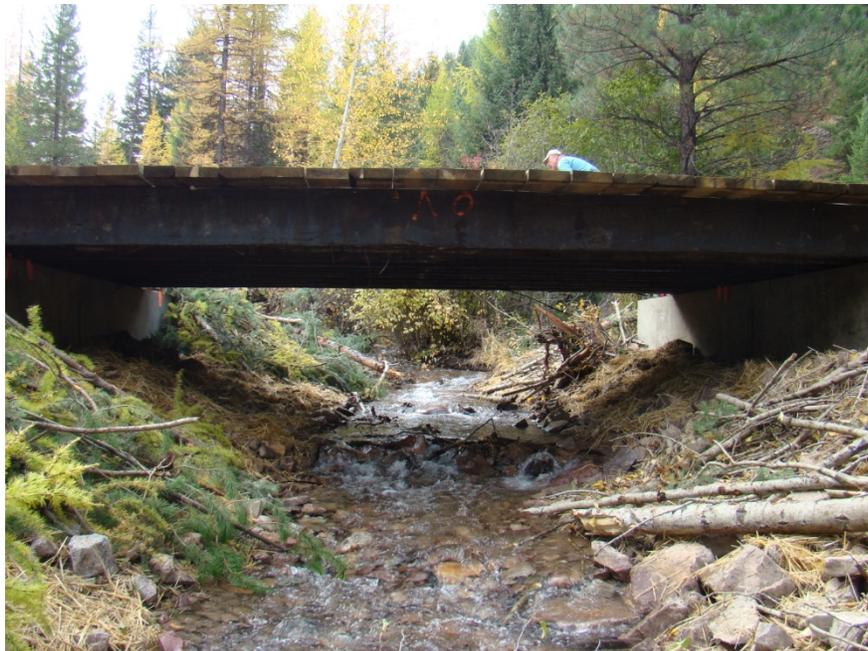
Historic undersized culvert on Bear Creek near stream-mile 2.2 replaced with a free-span bridge in 2011.
